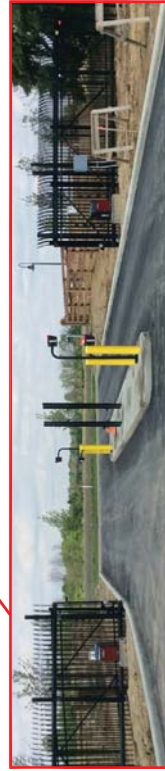
8' Tall Steel Security Entrance Gate (Ameristar AEGIS II)
