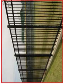
8' Tall Steel Perimeter Security Fence (Ameristar AEGIS II)
